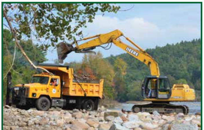
Working against the river – Heavy equipment raises the river bank, cuts the river off from its floodplain (where flood energy is naturally dissipated) deepens the channel, destroys fish and turtle habitats and directs more destructive flood energy downstream, thereby threatening homes and infrastructure there. Photo © Dan Plumley
