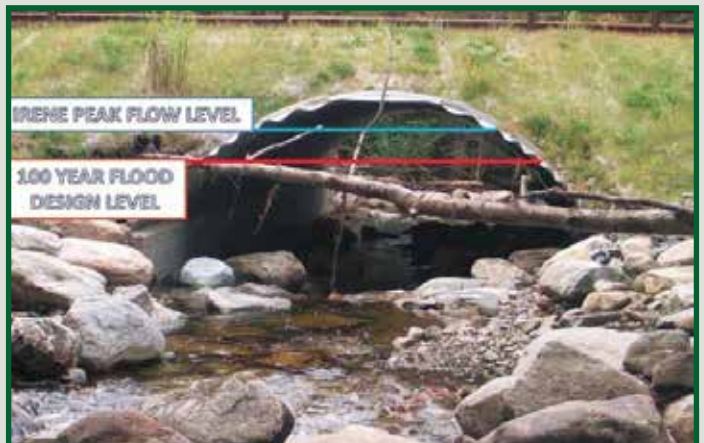
New arch culvert showing height of 100-year design flow in red and height of Tropical Storm Irene flood level in blue. Photo © Brian Austin, Green Mountain National Forest.
