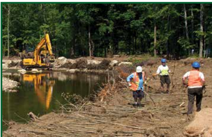
Working with the river – Streambank revegetation and riparian habitat restoration project along the East Branch of the Ausable River. These activities restore resilience to erosion while maintaining river-floodplain connection, thereby allowing flood energy to naturally dissipate within the floodplain instead of directing it all downstream. Pool-riffle habitats within the river maintained for trout populations and wood turtles. Photo © Ken Rimany
