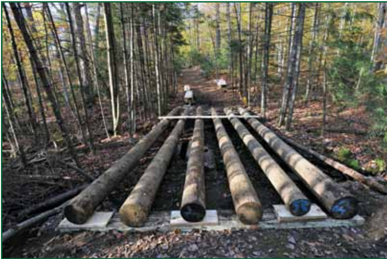
12-ft. snowmobile bridge is part of the newly constructed Seventh Lake Community Connector snowmobile trail in the Moose River Plains Wild Forest. Photo by Ken Rimany
